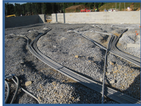
Figure 1.3: UG Electrical Rough-Ins
